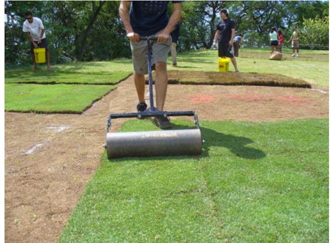
7. Lightweight rolling after sodding
