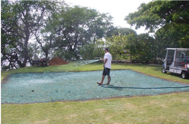
5. Application of hydromulch after stolonizing
