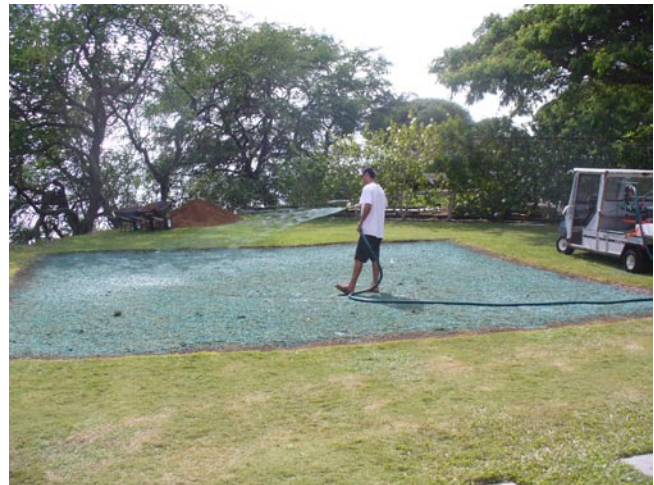
4. Application of hydromulch following stolonizing
